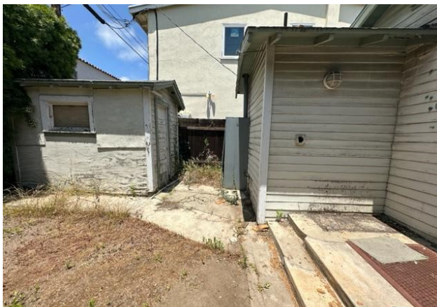
Storage Shed & Side Yard Garden
